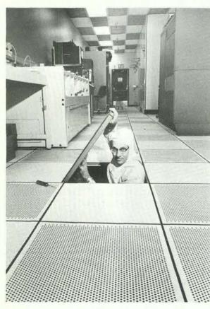
CHARLIE BARNES (2141) solves one last water leak under the floor of new clean room area in Bldg. 870. Filtered air flows constantly from ceiling to floor to provide super clean environment for the fabrication of IC devices.
